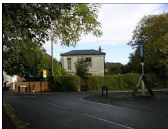
109 Obelisk Road – Original windows replaced with upvc units.
