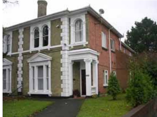
60 Portsmouth Road – Side extension clashing with the symmetrical proportions of the original building
