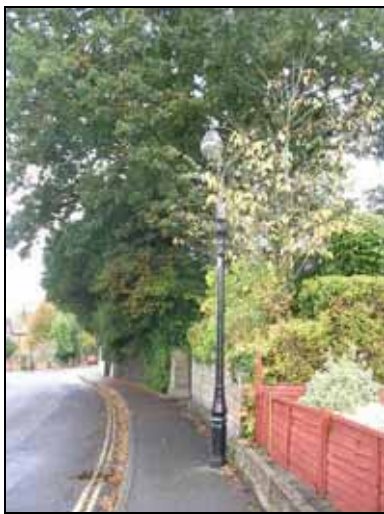
Oak Road – Cast-iron lamp column
