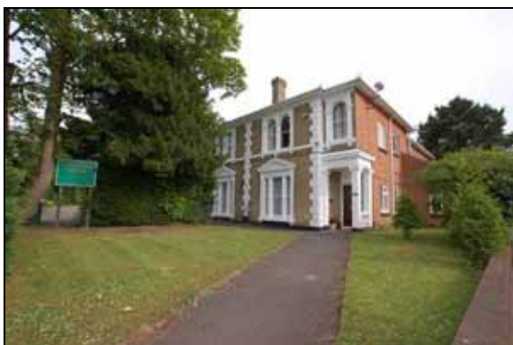
60 Portsmouth Road - Flats
