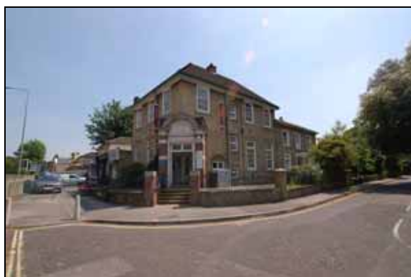
Woolston Library – Corner of Portsmouth Road and Oak Road
