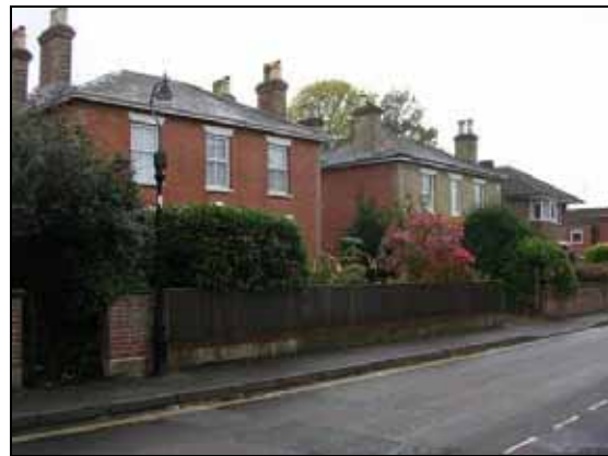
Mid to late Victorian villas on Oak Road
