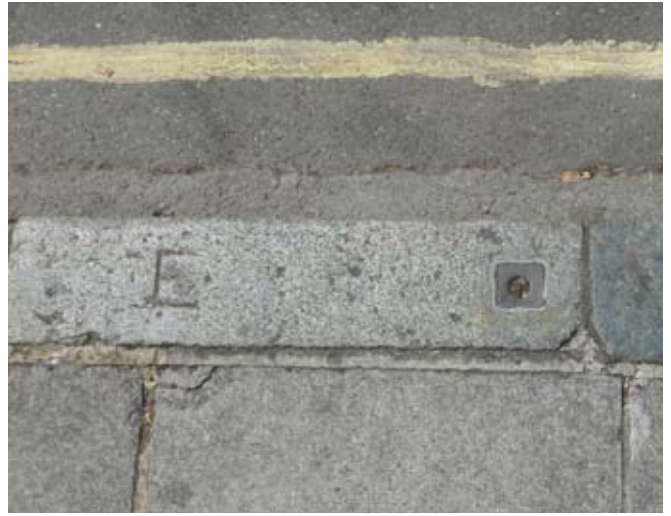
Granite kerb stone and steel socket used to hold up a shop front canopy, Oxford Street
