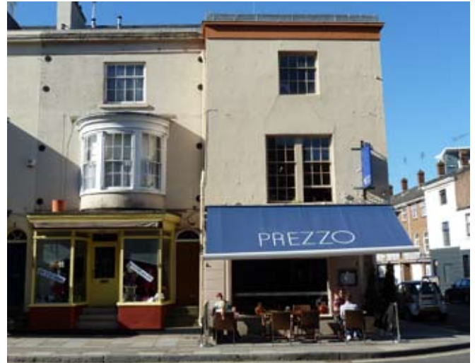
Plain rendered facade and intact shop front, 25 Oxford Street
