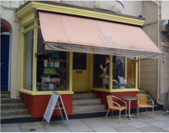
Intact historic shop front, 24 Oxford Street
