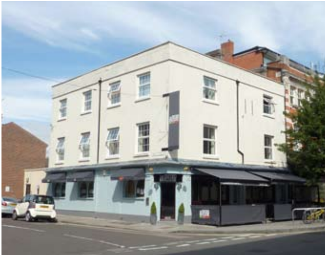
Simple stuccoed corner building, Oxford's Brasserie, Oxford Street
