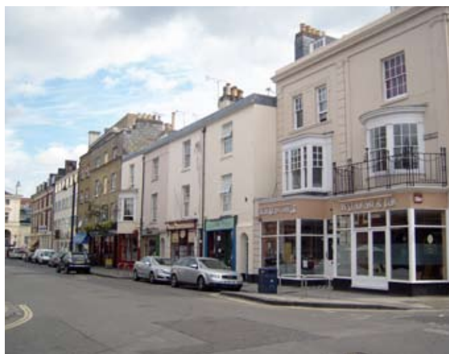
Mixed uses along Oxford Street
