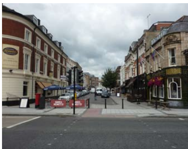
View along Oxford Street from where it is stopped off at its junction with Terminus Terrace
