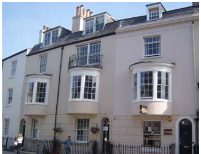
Fine distinctive semi-circular bow windows, Oxford Street
