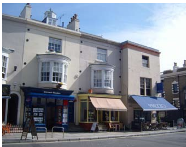
Early-to-mid-nineteenth century town houses converted into shops, Oxford Street
