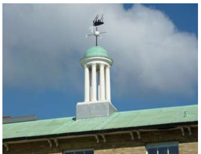
Copper roof and attractive central cupola with feature weather vane, Bowling Green House
