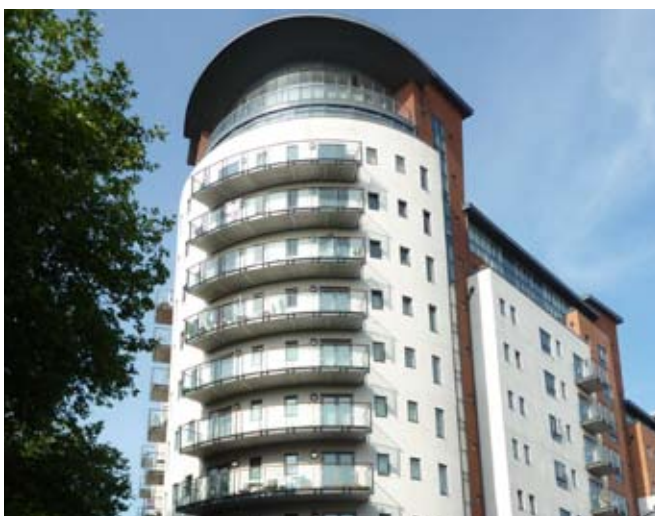
Out-of-scale and 'national' style Oceana Boulevard, Briton Street/Orchard Place
