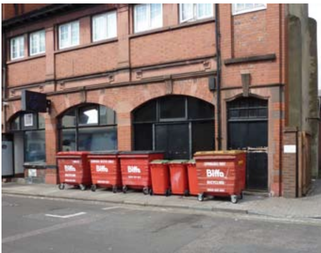
Commercial waste bins on the footway are a visual nuisance and obstruction, John Street
