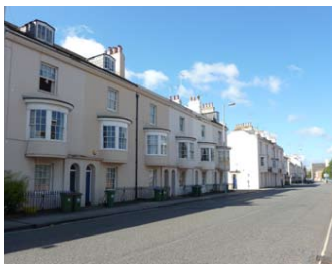
Nineteenth century terraced town houses, Bernard Street
