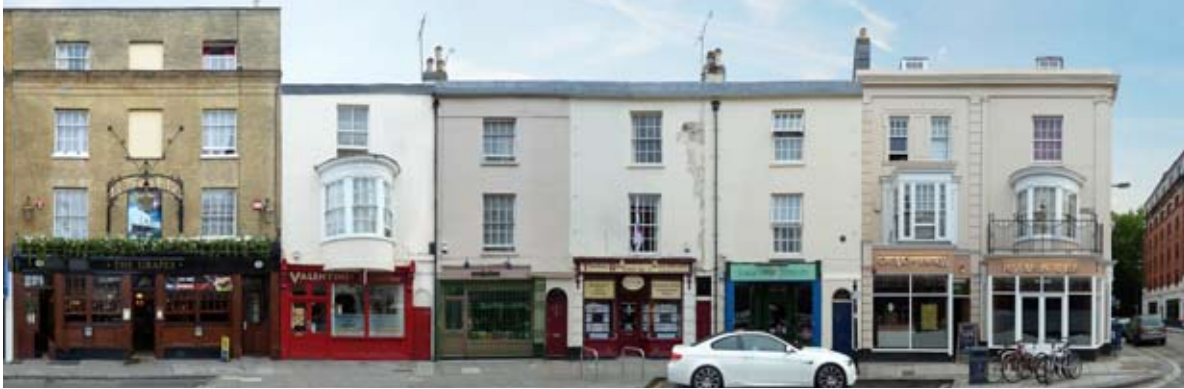
41-43 Oxford Street Grade II Listed
