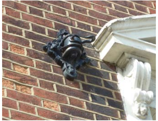
Cast iron tram rosette on the wall of The Court Jester public house, Terminus Terrace
