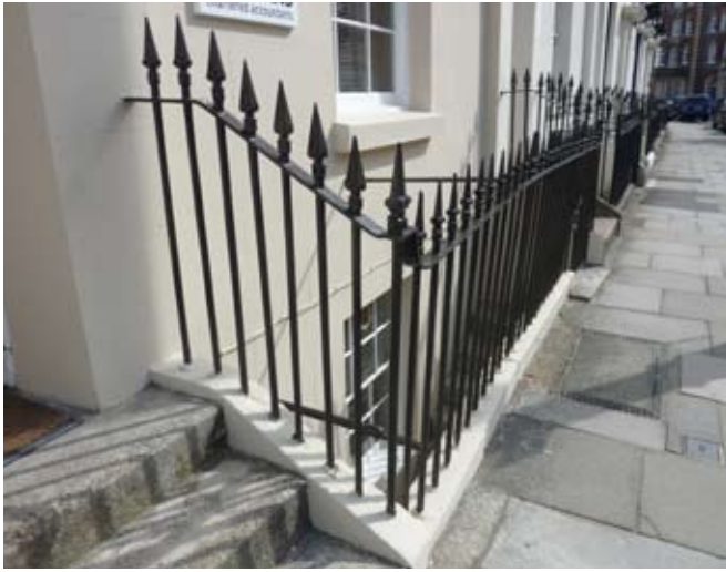
Attractive cast iron railings with spear heads defining the threshold to the property, Oxford Street
