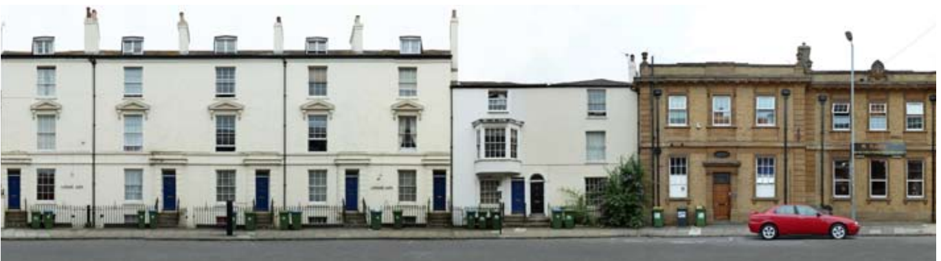
10-1 Latimer Gate, Bernard Street Grade II Listed
