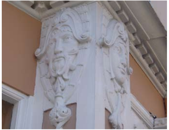
Decorative mouldings, 48-49 Oxford Street
