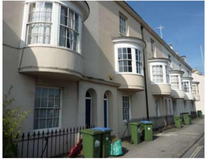
Wheelie bins on the street undermine the quality of the buildings and overall townscape
