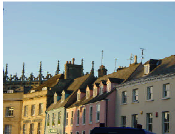
The roofscape is a particularly important aspect to be sensitively treated as it can add interest through variety
