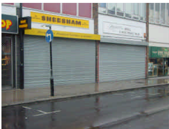
Shutters should be internal, and of the open lattice type, to avoid blank frontages predominating at night
