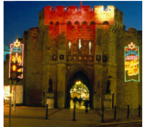
Flood-lighting should be used to enhance the Town Walls at night (© Joe Low)
