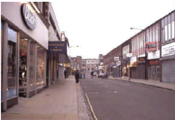
East Street highlights the need for stronger control of the clutter and obtrusiveness that shopfronts can cause
