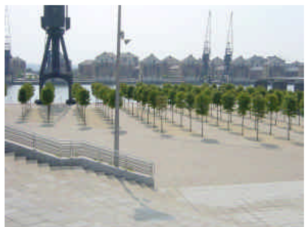
A contemporary mix of hard and soft landscaping in London Docklands
