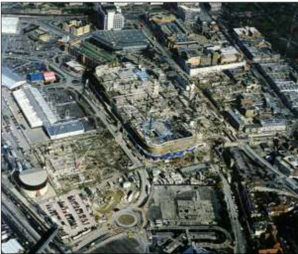
Development work on West Quay Phase 2 (Shopping Centre) March 1999
