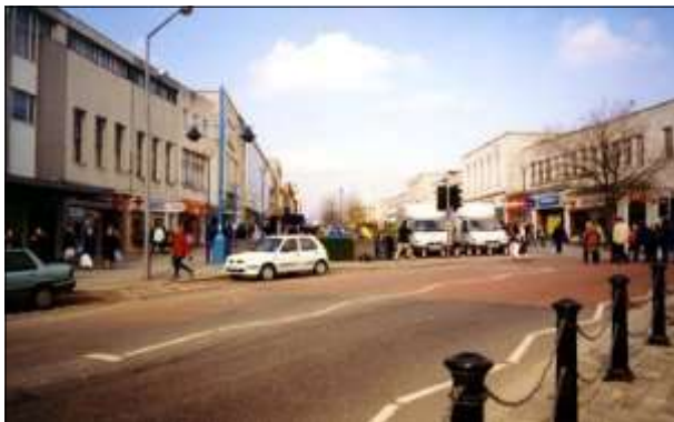
Cross city traffic conflict with the north south pedestrian routes at key locations.
