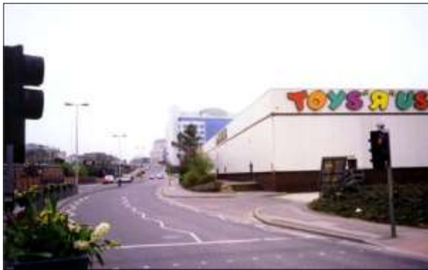
2 The Western Esplanade and Civic Centre Road offer a visually poor gateway into the city.
