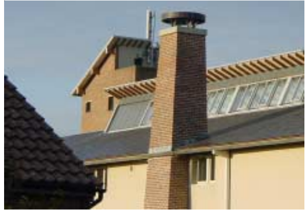
An articulate way of juxtaposing roof planes and chimney ventilation.
