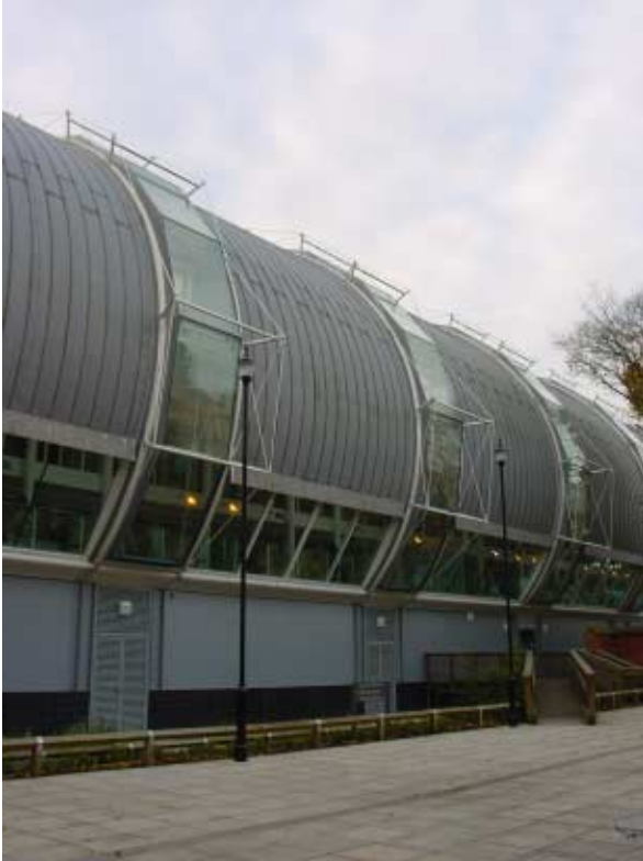
An innovative approach to façade design where the roof becomes part of the elevation - new Magistrates Court - Southampton.
