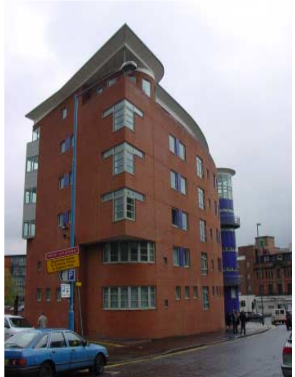
A brick clad concrete framed building - Birmingham.
