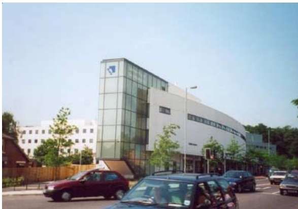
The façade facing the road is emphasised horizontally by the transformation of a regular plan to a sweeping of render and strip windows - Southampton University.
