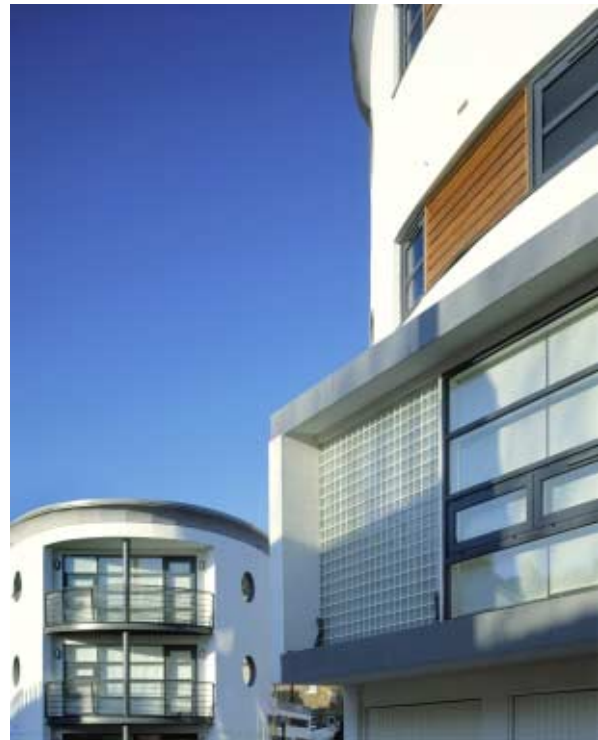
Balconies to the left of the photograph are designed integrally as part of the form of the building. The strong frame to the windows on the right emphasises the piano nobile - London.
