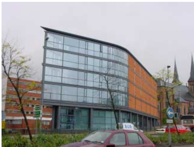
A steel framed building with brick panels and glass façades - Birmingham.
