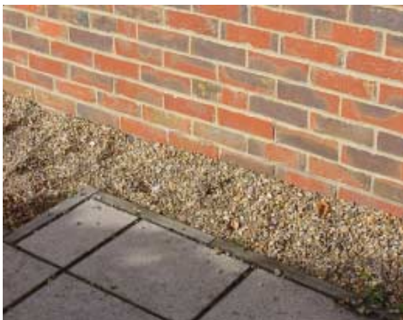
A gravel bed adjacent to the brick wall prevents splashback.
