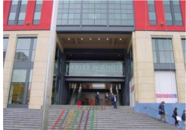
The two storey recessed entrance to this mixed development gives an impression of grandeur which is further enhanced by the stepped approach - Birmingham. Ramped approaches are also provided.
