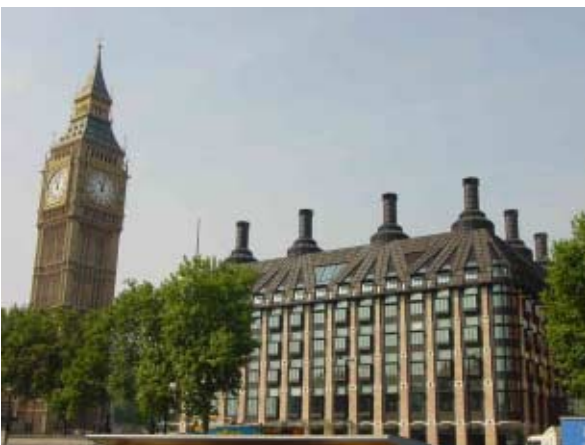
Portcullis House, London, is naturally ventilated.
