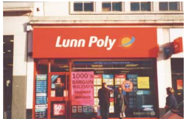
This fascia is too large and the colour too dominant for the shop size, although the red framing members are acceptable.
