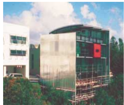
This live/work building in Auckland successfully uses an understated area of red to create a visual target.
