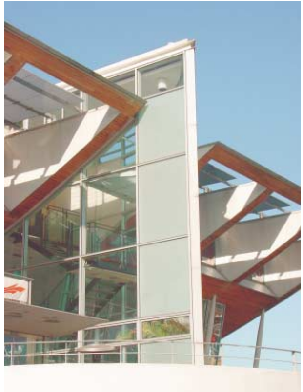
Glazing panels on the 'prow' of the Harbour Lights Cinema are proportioned according to the Golden Ratio. This is accepted as the rectangular shape with the most harmonious proportions. It's sides have the ratio of 1 : 1.618.
