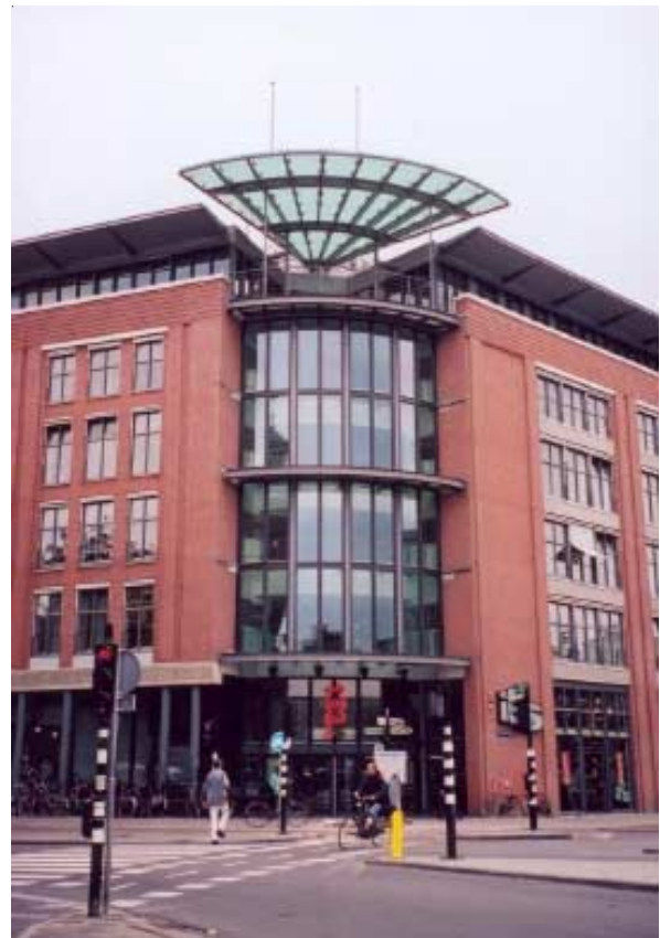
In this department store, the roof plane is emphasised by deep overhanging eaves, and the set back of the top storey. The proportions of the glazing on the corner and glazed canopy emphasise the entrance to this department store in Amsterdam.
