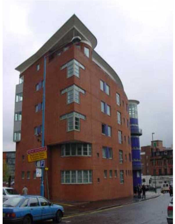
A brick clad concrete framed building - Birmingham.
