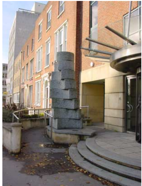
An ingenious use of sculpture forms the pivot for a ramped approach. A radial glass canopy embellishes the entrance.
