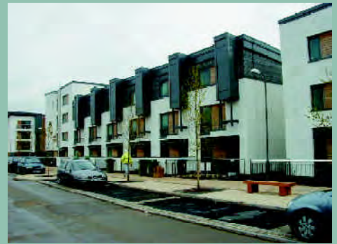
The front boundary walls of this development also provide natural ventilation to the underground car park - Chapel, Southampton
