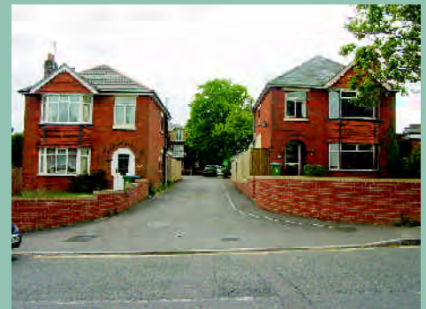
The design of this access to a backland development is sparsely detailed and does not make an attractive approach
