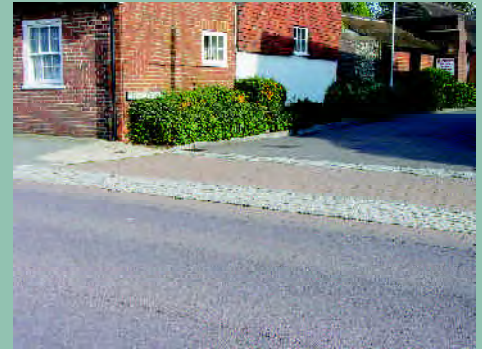
A footpath is demarcated in pavers and setts across an access to a backland development - Petersfield
