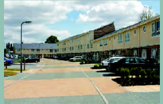
A shared surface for vehicles and pedestrians reduces traffic speeds - Mason Moor, Southampton
