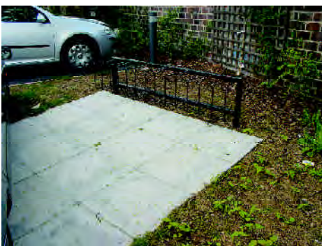
Cycle parking facilities for visitors should be provided alongside visitor parking spaces and kept accessible at all times. The surrounding areas of landscape should be easily accessible for maintenance, unlike in this photo.
