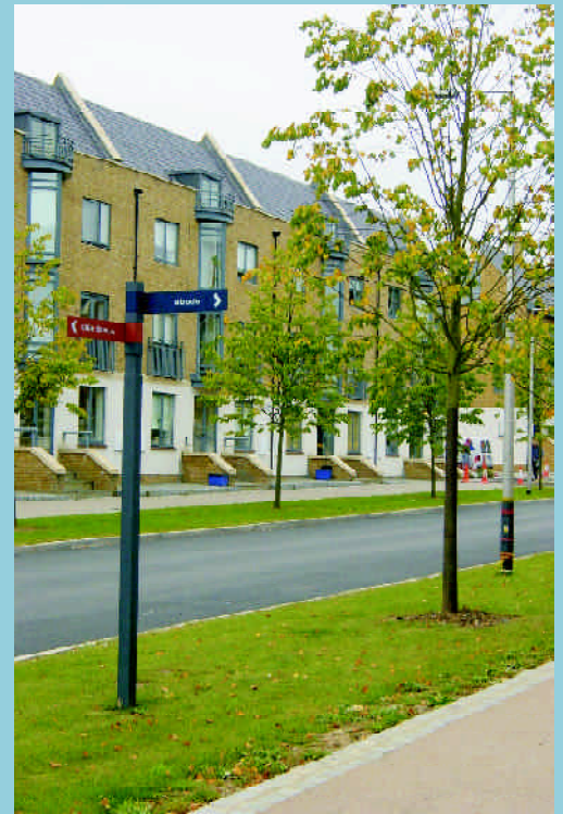
These town houses have no private soft landscape space in their front curtilage; instead an attractive boulevard of street trees has been planted - Harlow
