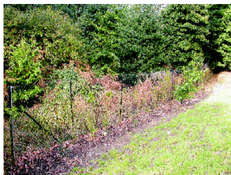
Suitable protection, such as this chain link fencing, should be installed on a site to protect existing habitats, such as badger setts and 'badger corridors' to facilitate movement
