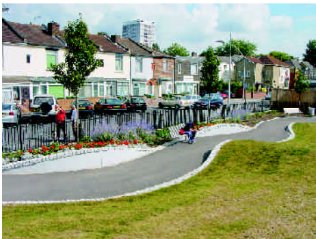
A new 'pocket park' has been created on previously derelict and under-used land - Northam Home Zone, Southampton
