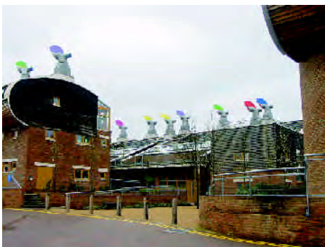
The work unit elevations are in the centre of this photo and have a grass roof providing amenity space for the house on the opposite side of the street - BedZed
