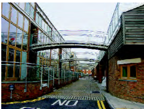
The bridge access to the grass roof of the work units form an attractive arcade to the street - BedZed
