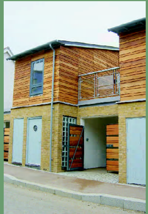
Narrow plots that front onto and back onto a street can be developed at both front and back giving potential for separate accesses, such as this 'back of pavement' development - Harlow
