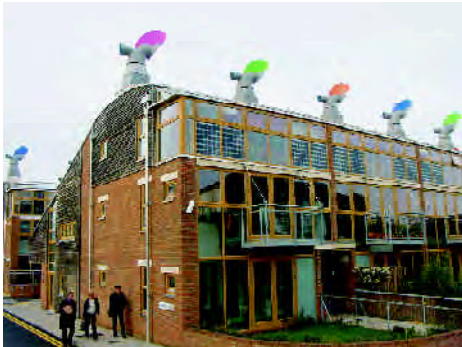
This housing has been designed with integral work units accessed directly from each dwelling. The work unit is on the left of this photo - BedZed
