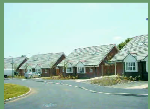
Mobility houses, houses offering easy access to people with mobility disabilities, Southampton
