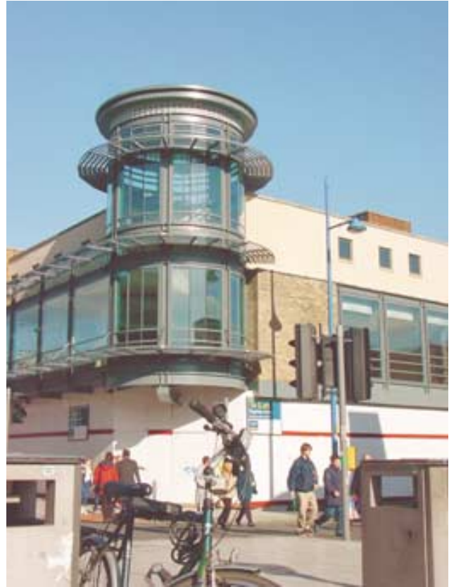
A successful corner feature on Above Bar Street, Southampton.
