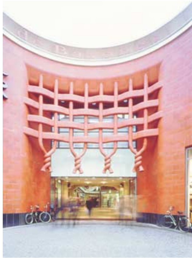
De Barones Shopping Centre, Breda, The Netherlands.
