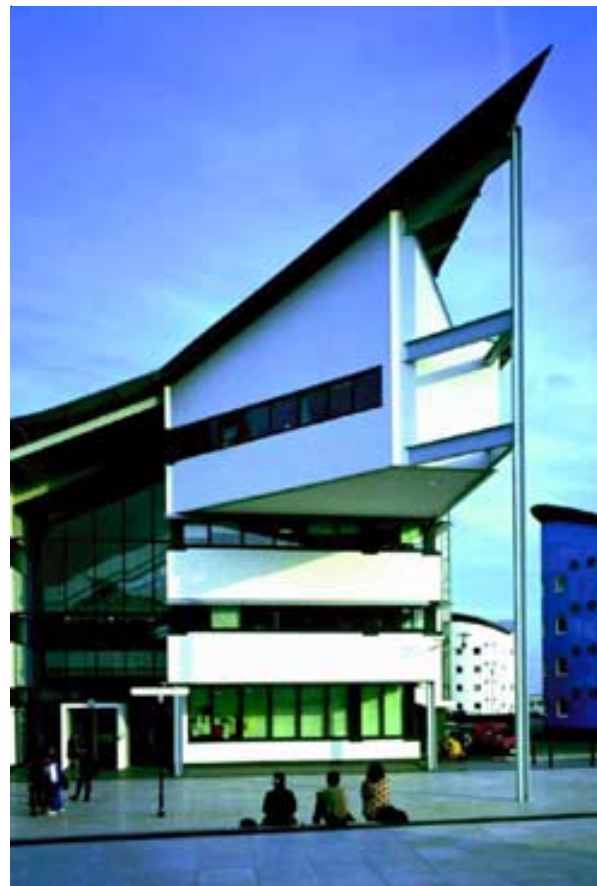
Corner feature - University of East London. © Edward Cullinan Associates
