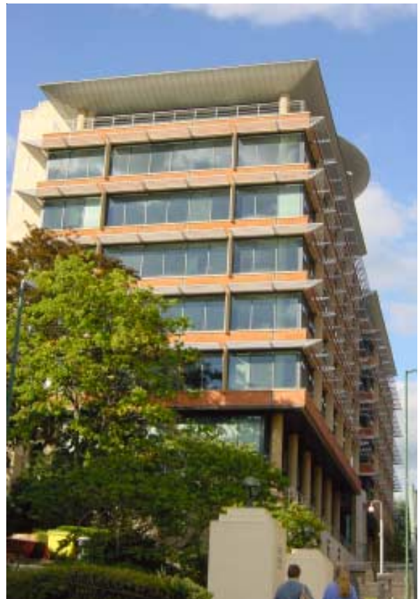
The shading devices on this building add interest to the skyline.
