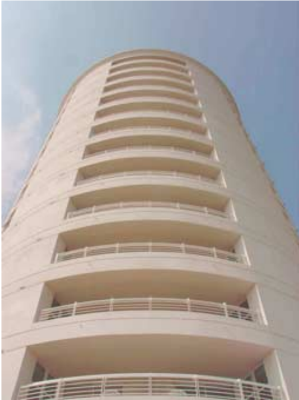
The dramatic presence of boldly detailed tall buildings can add greatly to the urban scene.
