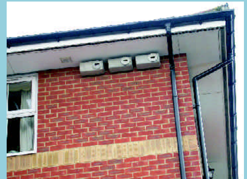
Nesting boxes for Swifts have been fitted under the eaves of this house to encourage swift numbers to try to prevent further decline of the species (25% in the UK since 1994)
