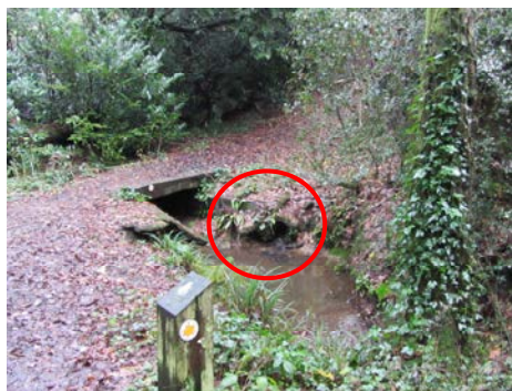
Photo 1: Surface water drain (circled) which discharges into the watercourse
