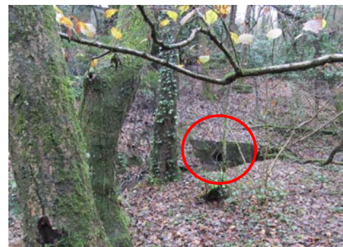
Photo 2: Surface water drain (circled) which discharges into the watercourse
