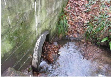
Photo 5: Culvert under a foot bridge
