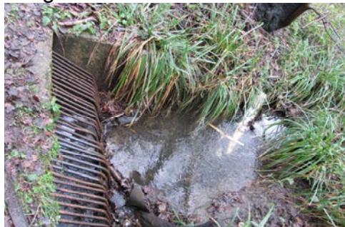
Photo 7: Trash screen where the watercourse enters the culvert under Lobelia Road
