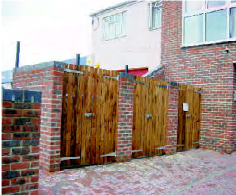
Full height storage areas are suitable for bins serving several residents
