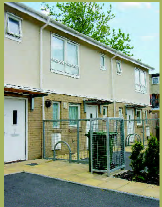
This galvanised metal fencing is attractive but is not designed to conceal the wheelie bin
