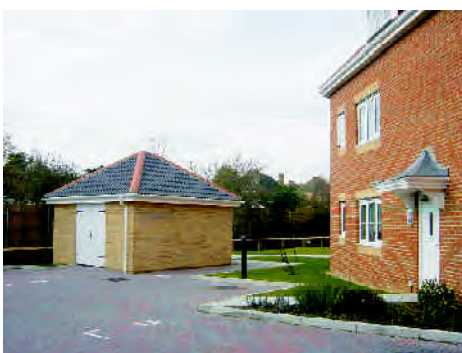
A free standing building provided for waste storage has been planned as part of the landscape and parking layout. However the side walls of the building could have been softened by evergreen shrubs - Fareham
