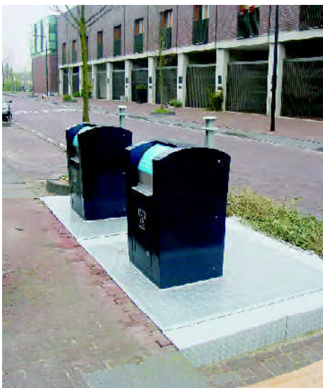
These underground waste storage systems in Amsterdam are an innovative way of containing waste discretely, however any proposals to use similar facilities should be discussed with the Waste and Recycling Manager
