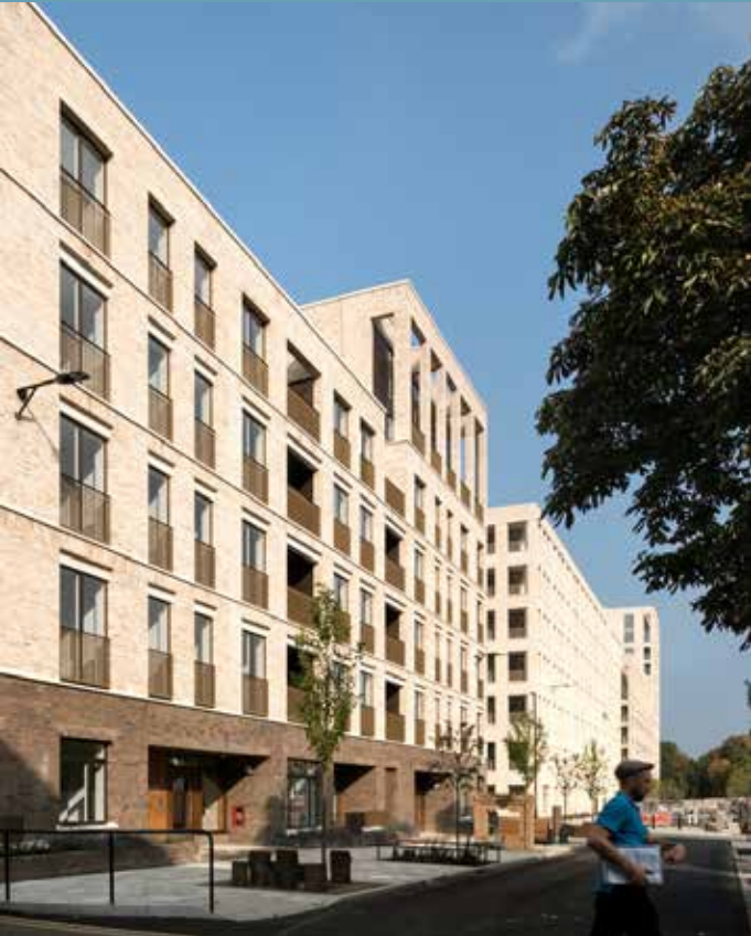
Housing - King's Crescent Estate, London
