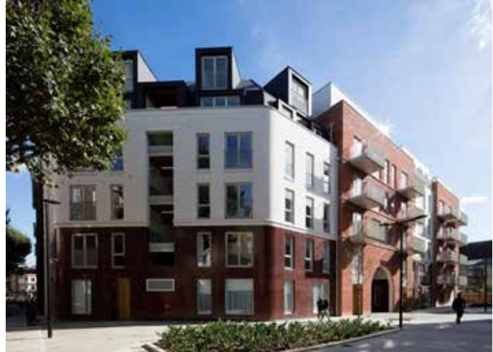
Residential - The Bourne Estate, Camden
