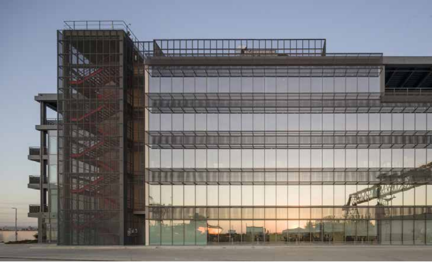
Port buffer - Shipyard Offices, Altinova
