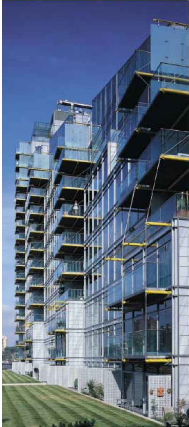
The mass and scale of large buildings can be successfully articulated by the emphatic detailing of the balconies and the varied skyline. Montevello, London - architect, Richard Rogers Partnership
