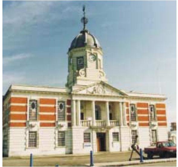
Some buildings in the waterfront area have Portland Stone or modern artificial equivalent horizontal bands set in red brick.
