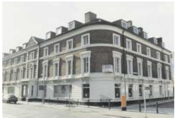
Red brick over a cream painted plinth with pronounced stonework is a common façade style in the waterfront area.
