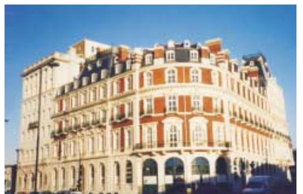
South Western House - Eastern.
