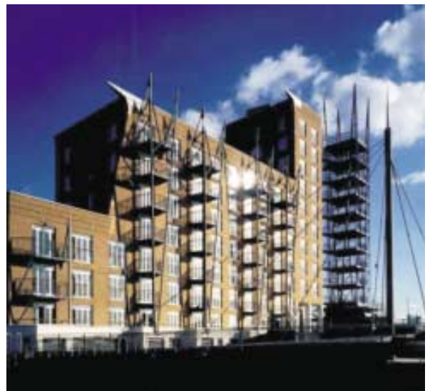
Dundee Wharf, Limehouse, London. The independent steel tower is a reference to the dockside travelling crane and this theme is further extended to the balconies in general; the pronounced 'V' shape being a reference to ships' loading booms (CZWG).
