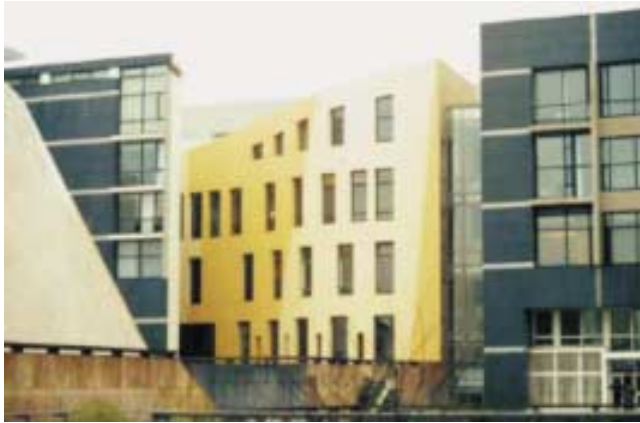
Wave form silhouette on a commercial building adjacent to Parc de la Villette, Paris.
