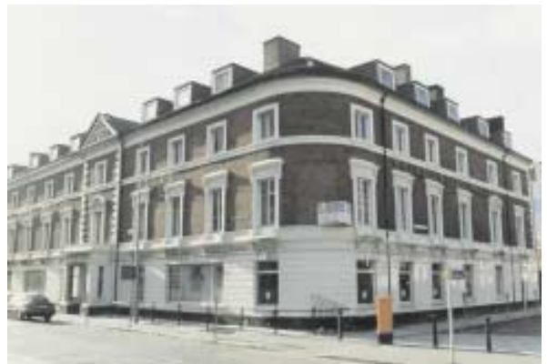
Red brick over a cream painted plinth with pronounced stonework is a common façade style in the waterfront area.
