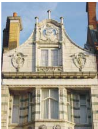
Building Detail - Old Town.
