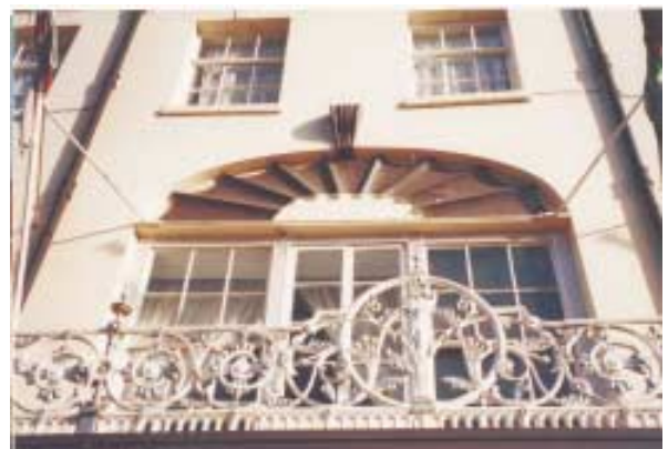
Building detail - Old Town.
