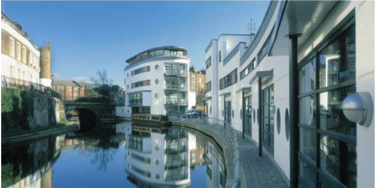
Above and left: urban chic at Lowford's Wharf in London. Subtle and sophisticated referencing of contextual form, shape, colour and rhythm. Copyright John Thompson and Partners and Benedict Luxmore.
