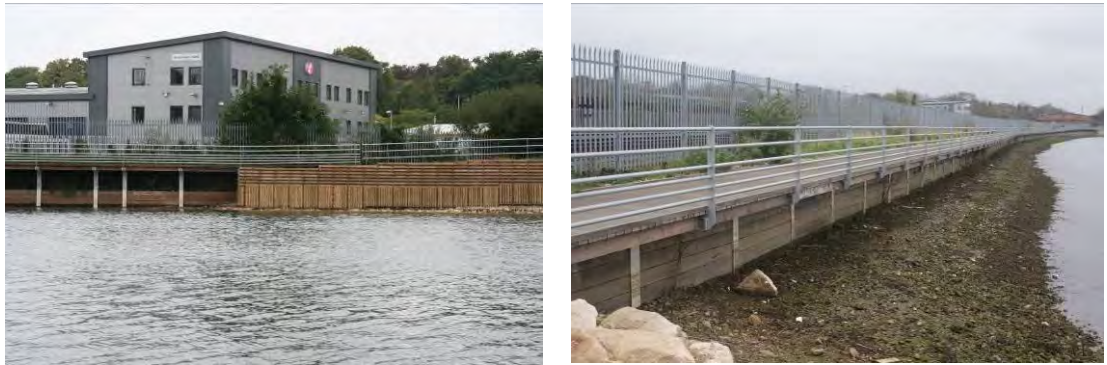
Figure 6-7. Photographs of the Bevois Valley frontage.
