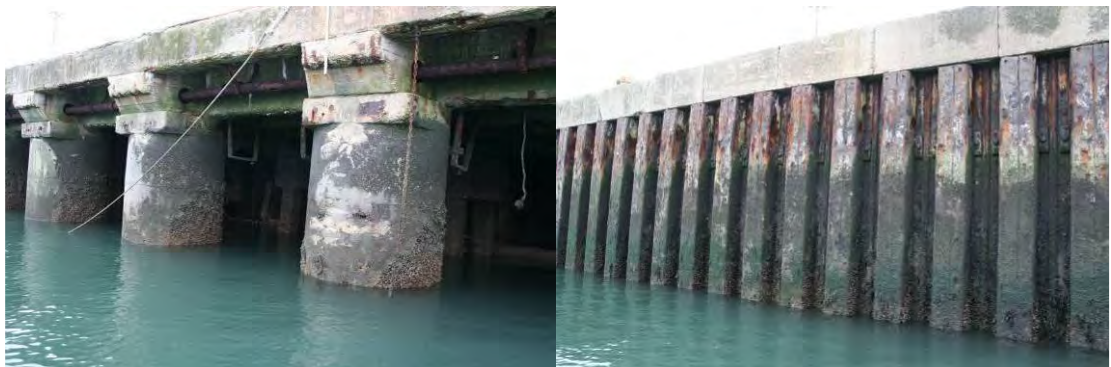
Figure 5-4. Quay walls along the Eastern Docks frontage
