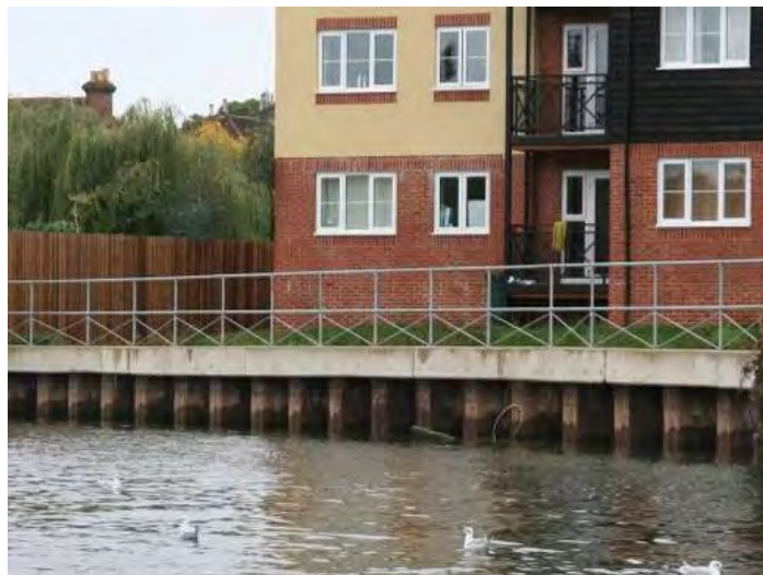
Figure 8-2. Steel sheet pile defences
