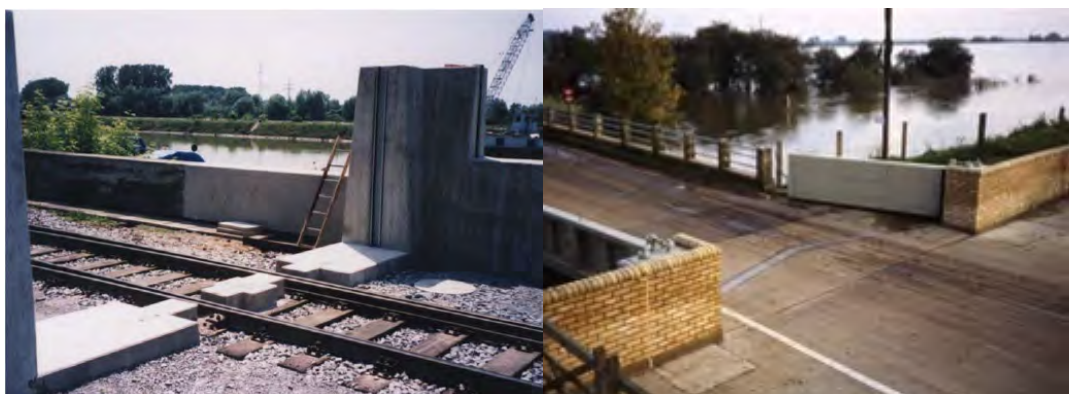
Figure 8-5. Demountable flood defence over a railway (left) – Courtesy of Bauer Demflood xi and (right) swinging flood gate across a road –Source: Environment Agency FCERM Fluvial Design Guide xii .
