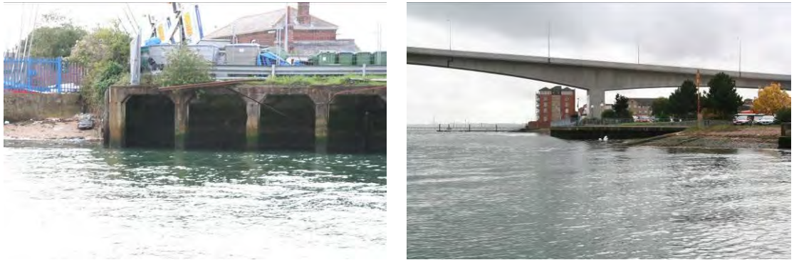
Figure 6-11. Photographs of the Town Depot frontage.
