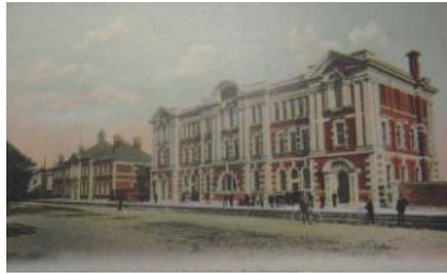
Figure 14. Post Office and Customs House, 1905
