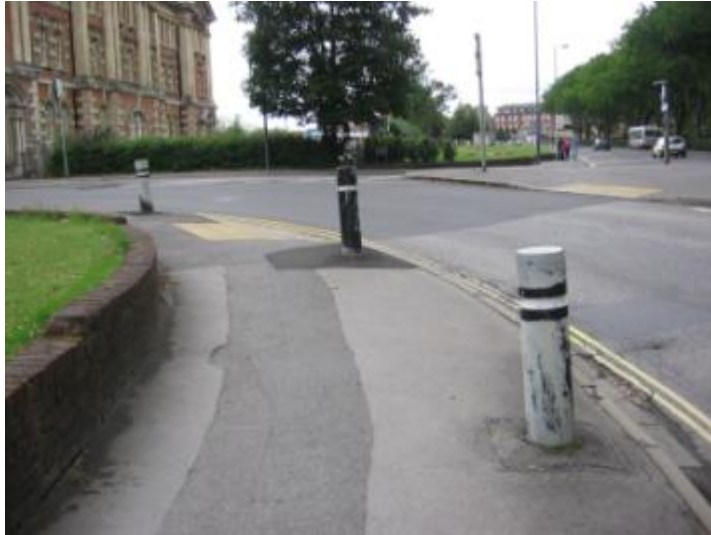
Figure 56. Dock Gate 4 bollards and crossing
