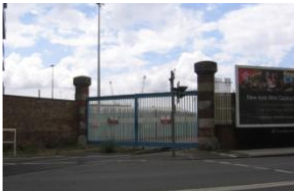
Figure 22. Railway gates and piers to south
