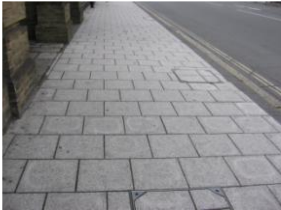
Figure 49. New paving, Canute Road Platform Road
