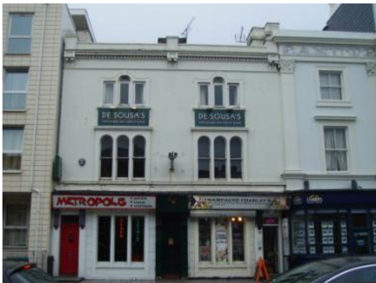
Figure 38. Nos 10-12 Canute Road
