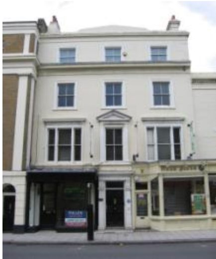
Figure 43. Nos 2-3 Canute Road
