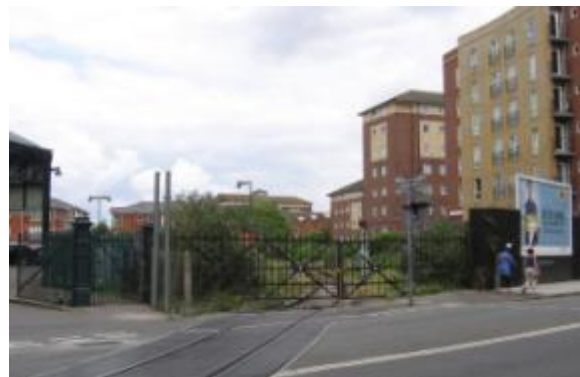
Figure 23. Railway and gates to north
