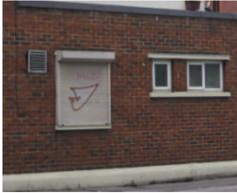
Figure 62. Security shutters, Royal Crescent Road Canute Road
