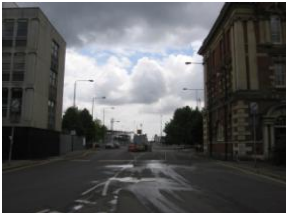
Figure 15. Dock Gate 4, view to south traffic
