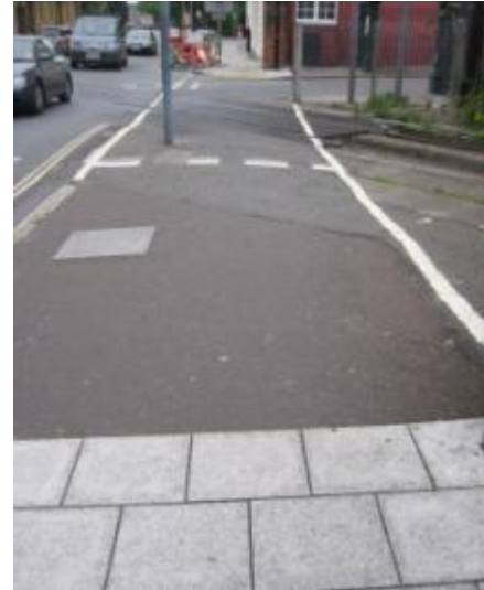
Figure 57. Pavement at railway crossing, Canute Road
