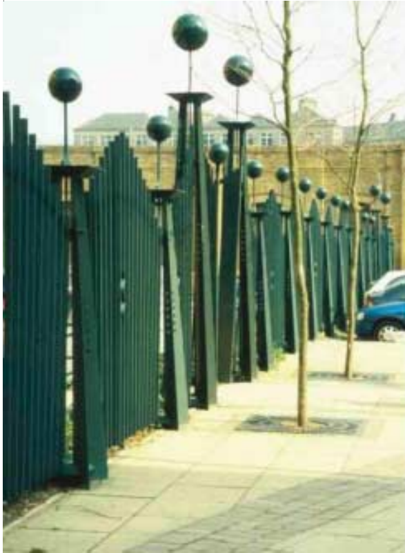
Railings - Inland Revenue, Bradford.
