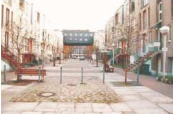
Purpose built shared surface street - Berlin.
