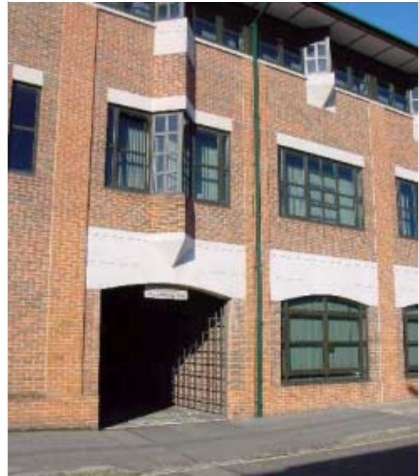
An excellent example of integration of a carriage arch into a building façade - Woollen Hall, Southampton.
