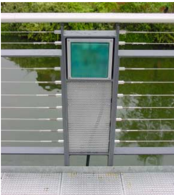
Integrated lighting detail.
