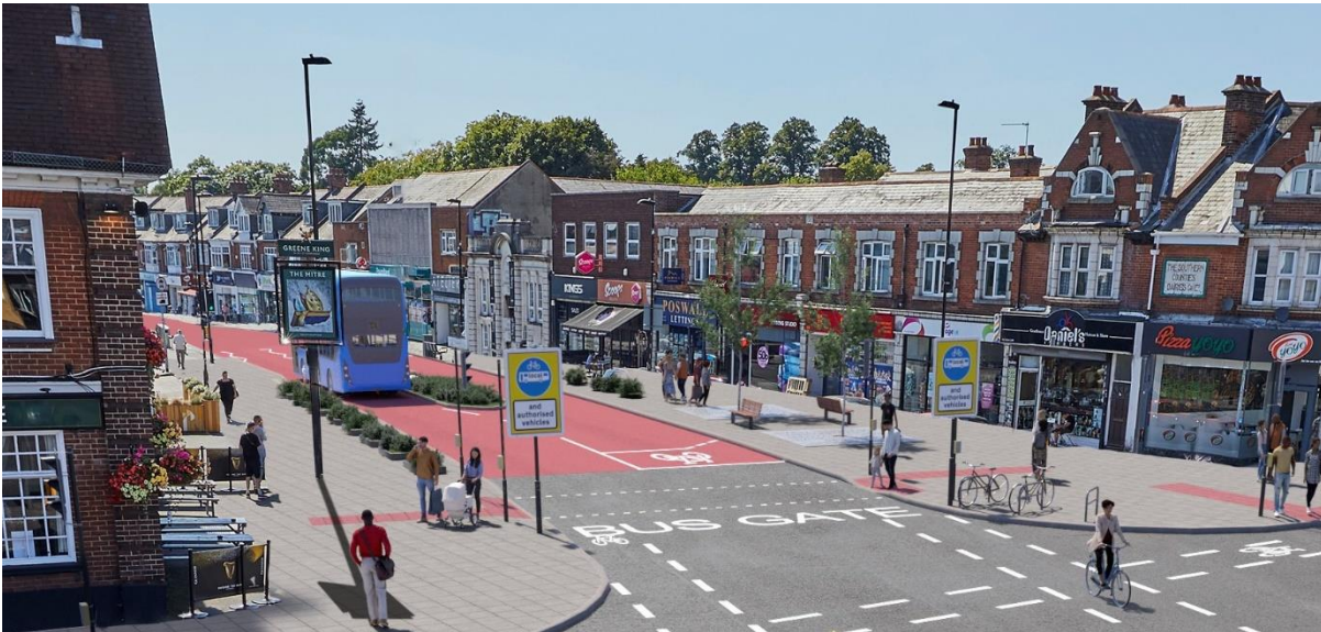
Figure 3 Portswood road scheme involving reallocation of road space to buses and cycles currently planned through TCF. One example of the scale of work being planned through the programme.
