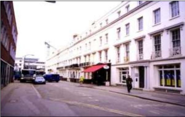
Portland Street provides an attractive western link to Above Bar
