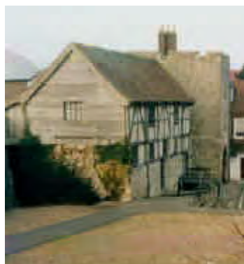
Westgate Square provides an ideal example of where the potential to make more use of some of the current open spaces of intrinsic special charm and character within the Old Town, exists
