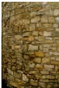
Many prestigious medieval buildings and the Town Walls, were constructed using stone from the Isle of Wight
