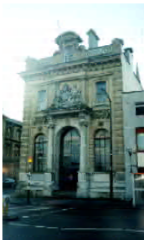
One of the many ornate banks within the Old Town, this example built using ashlar stone
