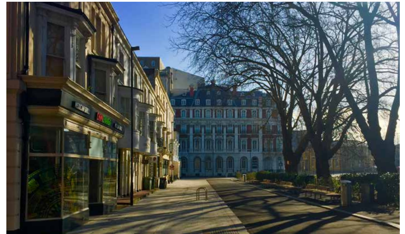
3 Street enhancements to Queens Terrace have delivered wider footpaths, new seats, tree planting and an extension to the existing park
