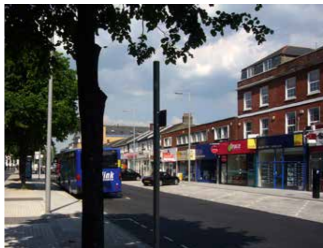
3 Public realm enhancements to London Road have stimulated a greater range of businesses and services, increased residential living, re-establishing this route as an important local high street
