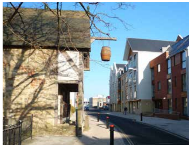
2 Details on an individual building can become important features which aid navigation within the city centre
