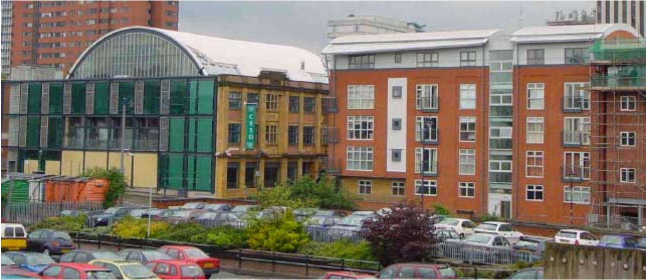
The scale and form of the new building on the right echo the design of the refurbished existing block on the left; Birmingham.
