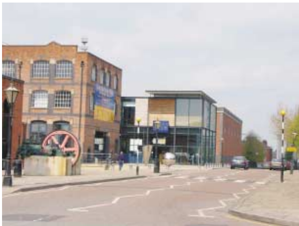
The Museum of Science and Industry in Manchester is a highly contemporary building that sits well against an old warehouse because it respects the form of the context. The result is rhythmical yet varied streetscape.
