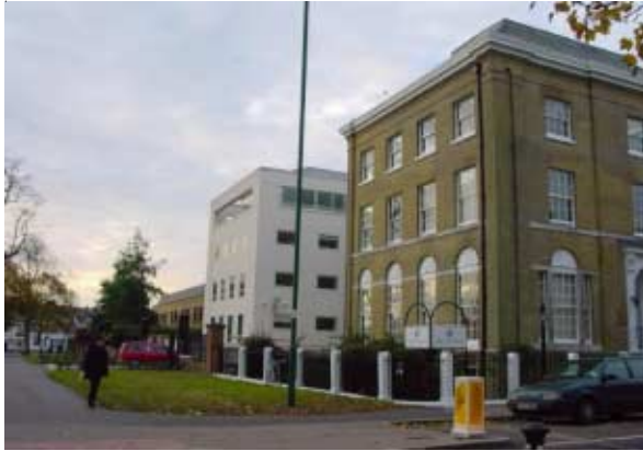
The scale of the rendered building respects that of the existing brick building - new Magistrates Court, Southampton.
