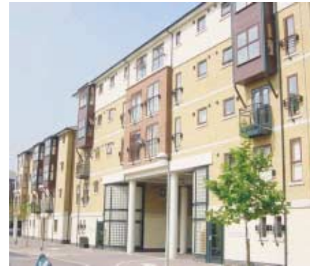
Access to the centre of perimeter blocks should be via a carriage arch to maintain street enclosure.
