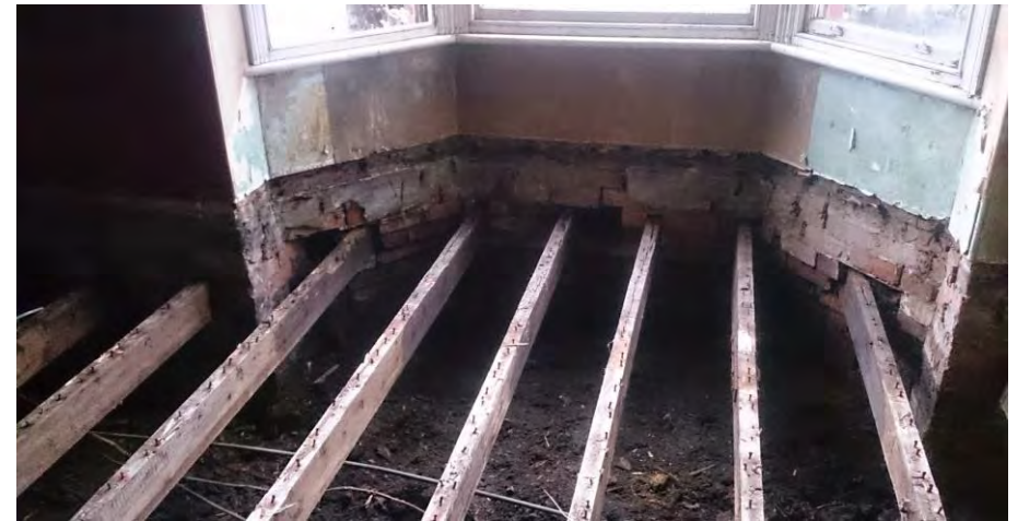
Achieving airtightness is possible in retrofit, but it is often necessary to strip back to the basic structure and perform basic repair work before methodically applying airtightness products and principles. Always consider risk of moisture and condensation. (Source: Eightpans)
