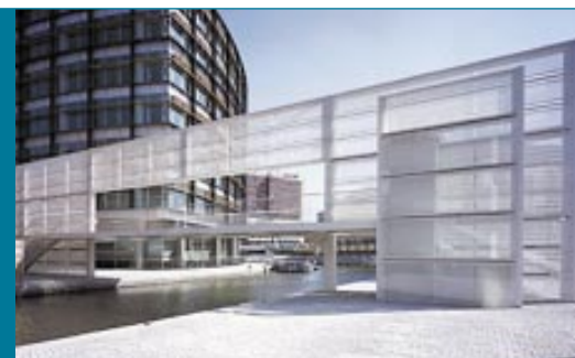
Langlands & Bell Paddington Basin Bridge 2004, London
