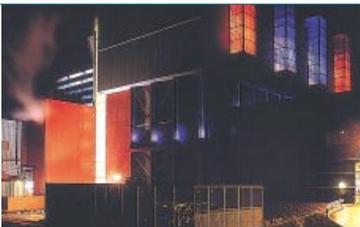
Martin Richman Energy from Waste Centre, Tyseley
