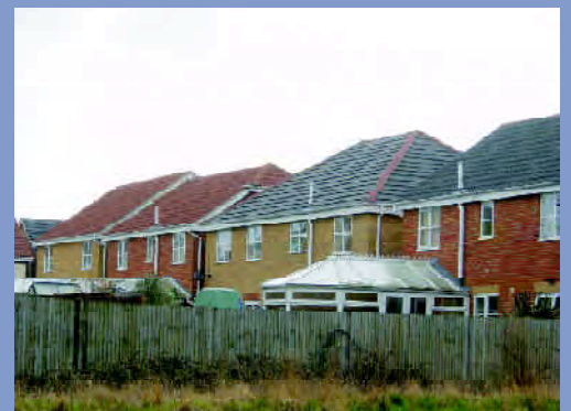
Exposed soil pipes to the rear elevations of these houses look unsightly
