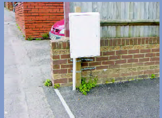
Meter cupboards should not be located in visually obtrusive places and where they are vulnerable to damage
