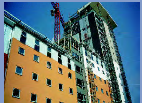
Off site pre-fabrication of units can reduce costs and construction time on site, however care must be taken that cladding materials are appropriate for the context and well detailed - Mercury Point, Southampton
