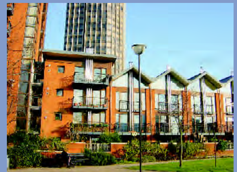
New development with a strong and positive visual impact can improve the local identity of a place - Coin Street, London
