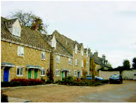
The building lines of this courtyard development line up with adjacent development
