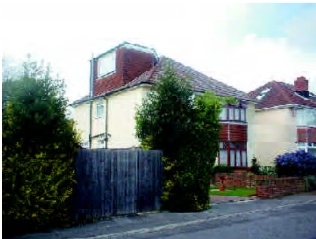
Dormer windows should not dominate the main roof form, nor should they be higher than the ridge of the main roof
