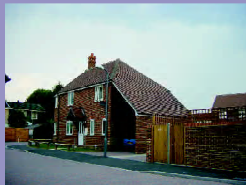
This carport has been sensitively designed using an extension of the main roof at the same pitch and with the same roof tiles
