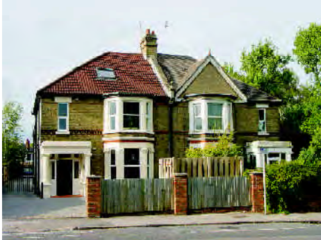
The removal of existing features, such as gabled roofs will be resisted. Roofs should be retiled with tiles of similar characteristics to the original ones
