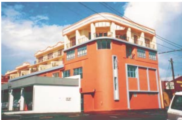
Conversion of a warehouse to residential use - Auckland.
