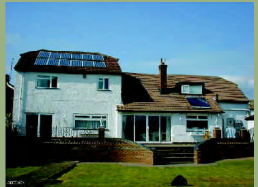
Dwelling fitted with solar water heating panels (right) and photovoltaics to the roof © Bre 2004
