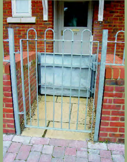
Flood gates fitted to boundary walls of 225mm thickness to provide resistance to potential flooding of individual terraces - Hythe
