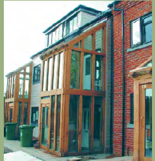
The two storey conservatory provides a thermal buffer; warming cool air before it enters the house
