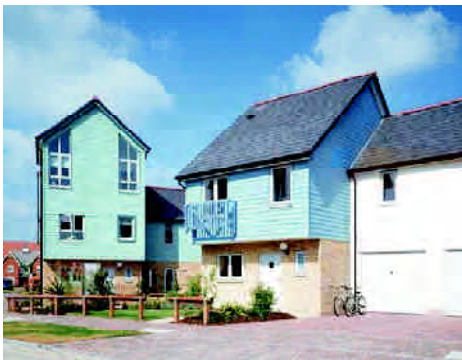
Ecohomes - award winning energy efficient housing; a joint venture project between Countryside Properties and SEEDA, St Mary's Island, Chatham Maritime, Kent - Developer: Countryside Properties Architect: Countryside Properties Architects with OSP Architecture © Countryside Properties
