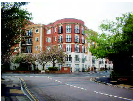
The combined heat and power plant in Southampton feeds these apartments in the Polygon
