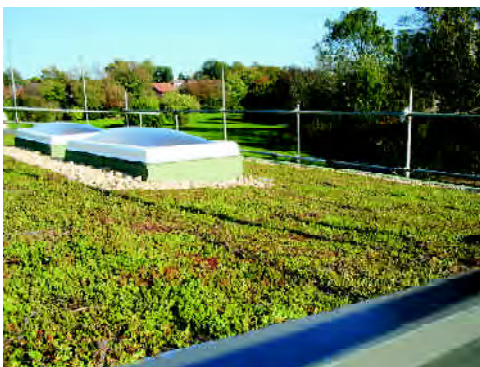
A green roof with sedum planting used on a public toilet block at Weston Shore, Southampton, designed by Southampton City Council Building Design Services
