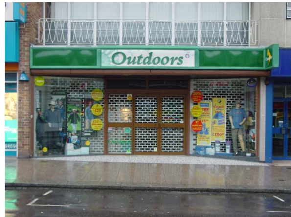
A well-designed security shutter that protects the shop's stock but retains a window display, allows views through into the shop and lets light spill onto the pavement.
