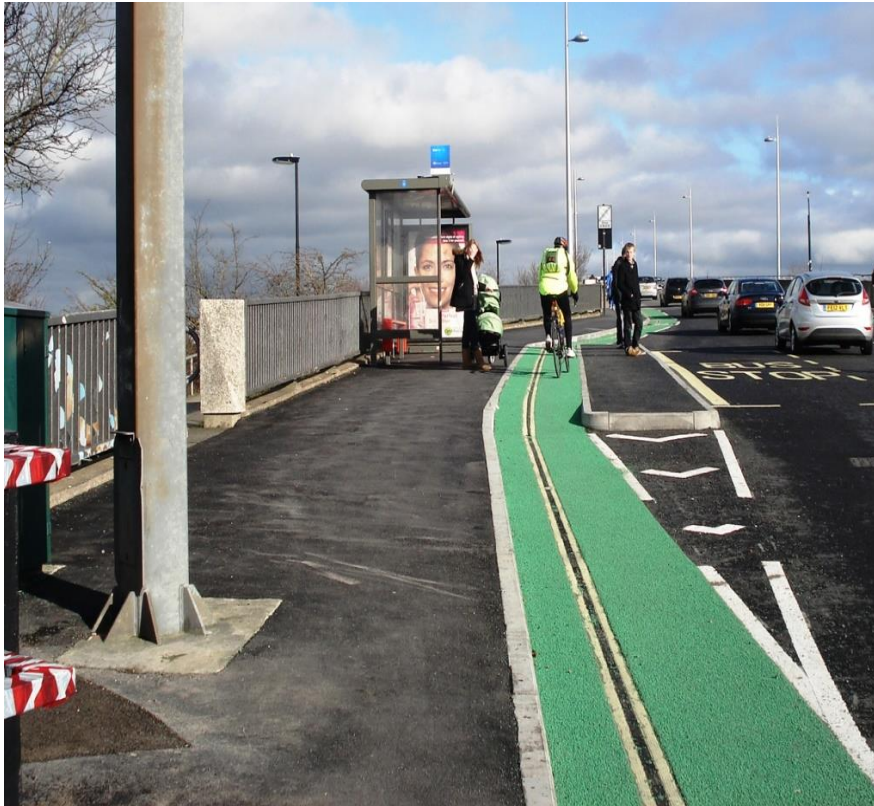
Figure 1 cycle lane on the Itchen Bridge
