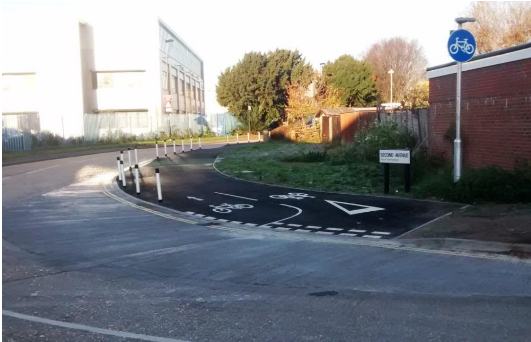
Figure 5 Photo of new off road cycle lane at Second Avenue, alongside Redbridge Road AQMA
