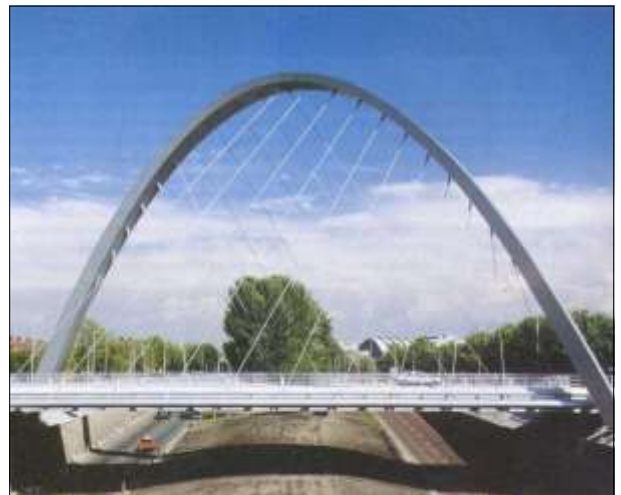
to reinforce connection with St. Mary's and the pedestrian link through to the Central Parks. Striking bridge link providing a strong gateway entry into the city centre, Hulme, Manchester
