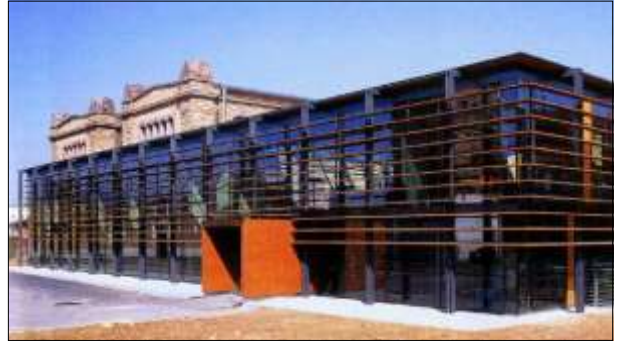
Pavillion style architecture - Landau City Library, Landau, Germany
