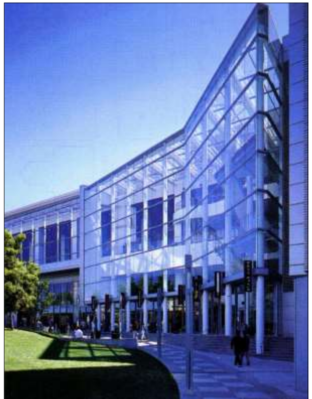
Glazed facades mark a permeable frontage to open space Metreon, San Francisco
