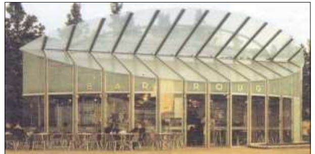
The central zone of the Above Bar precinct could be enlivened with a unique cafe building, Brindley Place, Birmingham
